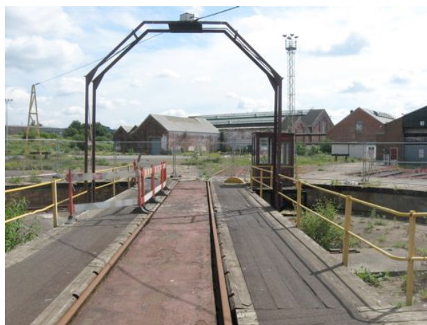
The one remaining locomotive turntable in the old Great Western depot at Old Oak Common in the north of the borough. The turntable pit is from 1906 when the depot opened. The large two-bayed building in the middle distance is the 'Factory', the Great Western's maintenance shed depicted on the cover of our last newsletter. The site now belongs to Crossrail.
