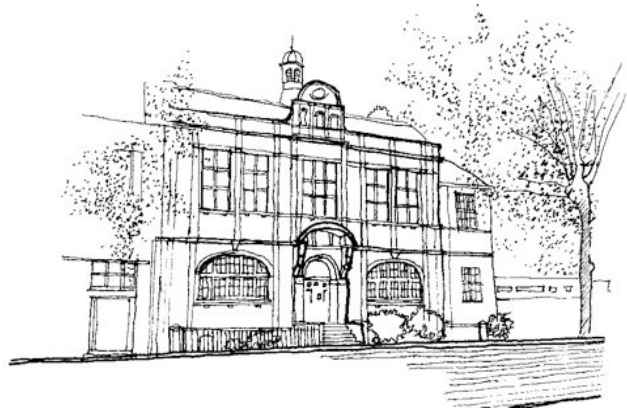
LAMDA, 153-155 Talgarth Road, designed by J. S. Quilter in 1894 for the Froebel Institute Training College
