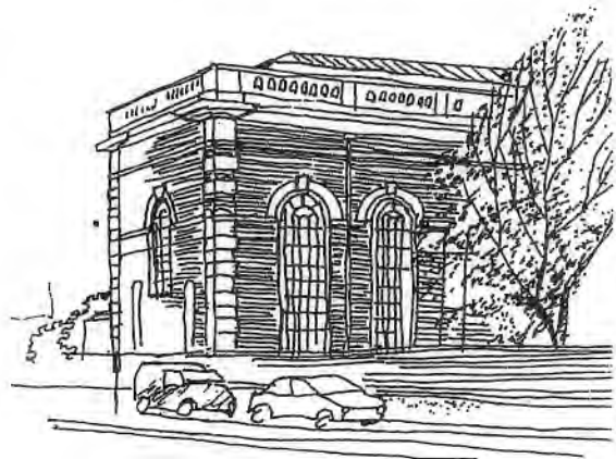
Hammersmith pumping station
